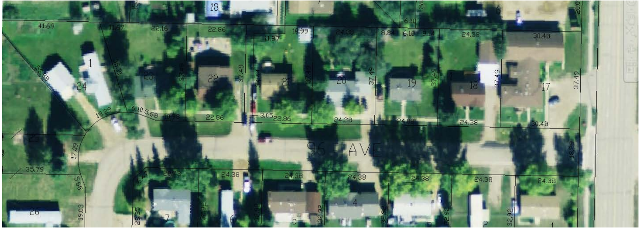
Aerial showing sidewalk on private property.
