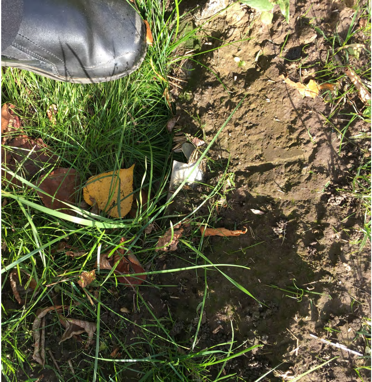
10010 and 10014 - 96 Avenue Access Culvert
